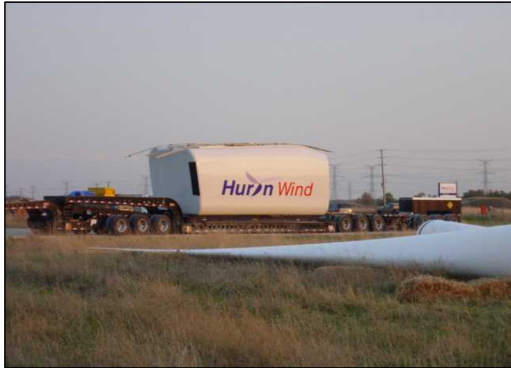
A 63-tonne nacelle arrives at the Huron Wind farm during construction in the fall of 2002. A partially assembled rotor is in the foreground to the right.
